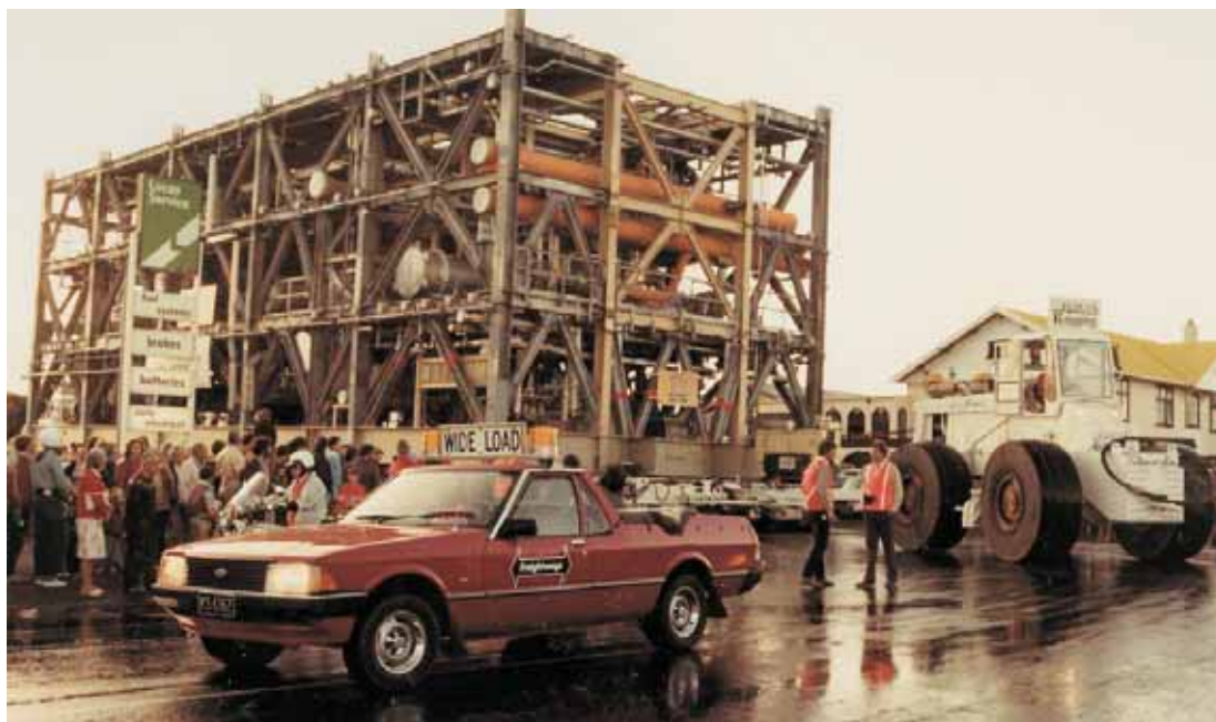
Figure 6: P0106 approaches Gill/Hobson intersection - the tightest corner on the haul route
