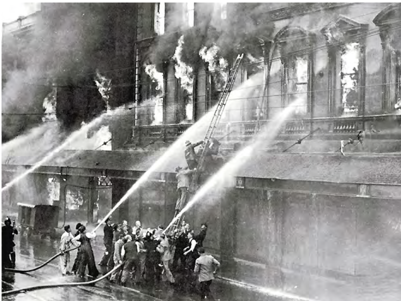
Figure 1.1: The worst fire disaster in New Zealand was the 1947 Ballantynes fire in Christchurch where 43 people died (photo courtesy of The National Library of New Zealand)
